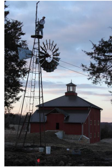
1920s Aeromotor being installed
