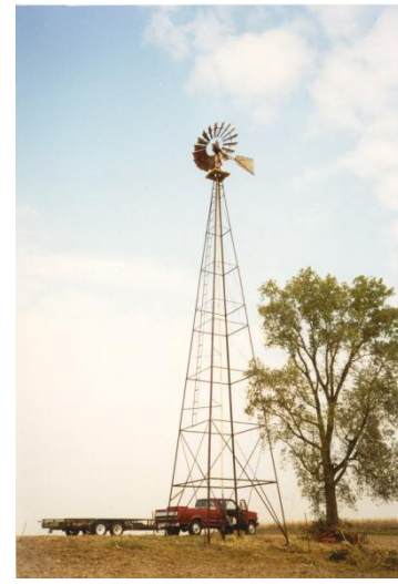
Rebuilt 8' Aeromotor & 60' Tower
