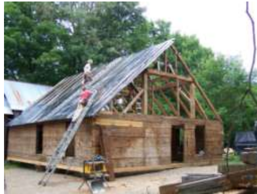
This is the building being reconstructed in the yard
