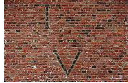
Clinker bricks used to form family initials TV 1700s Jan Van Hoesen house a Dutch house in upstate New York.
